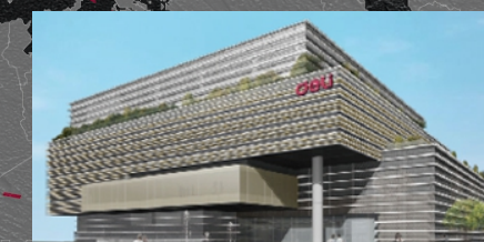
Ningbo Innovation Center
